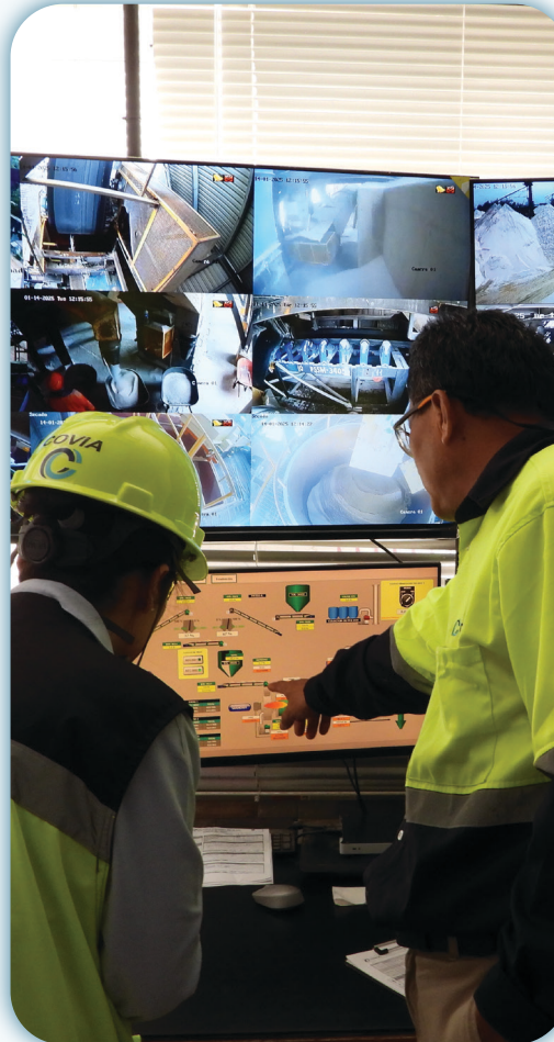
The Control Room (Ruben Peña)
