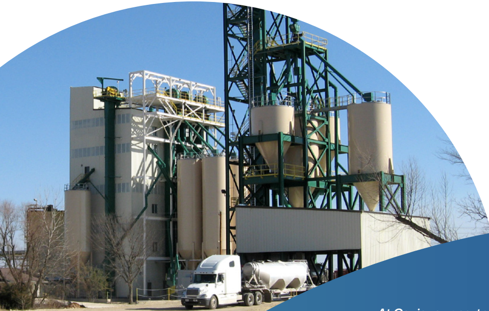
Photo of the loadout facility at our Roff, OK, site.
